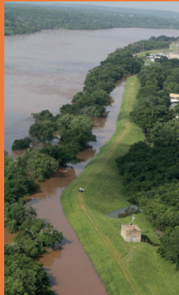
Tulsa Levee in 2019 Flood
